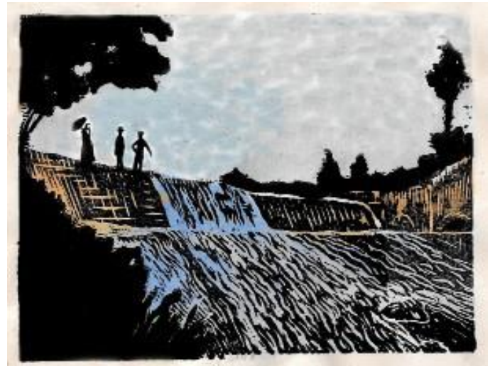
WB-8. The Flow Is Stemmed (The Plug Is Replaced)
